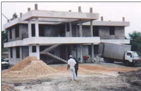
The hospital clinic at the Kibaha complex sponsored by WIPAHS under construction and nearing completion.
