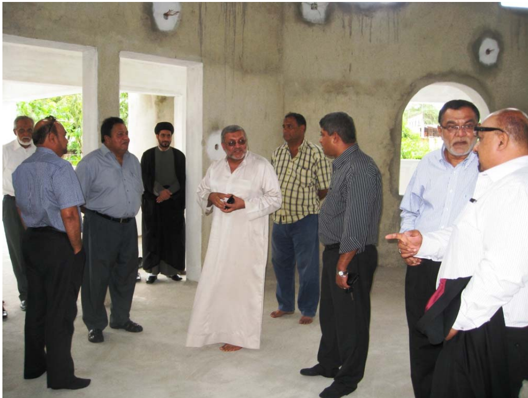
Top: The new Mosque in Nacala under construction. Above: The WF President, AFED Chairman and the delegation inside the Mosque, looking at the construction works. The Nacala Resident Maulana, Seyed Shazad Hussain was present during the entire visit, Similarly, Sheikh Dr. Muhammad Canani accompanied the delegation to Nacala for the visit.
